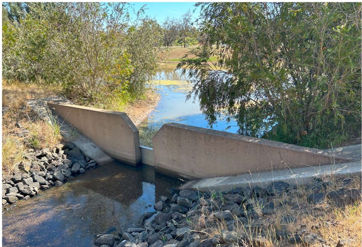
Figure 12 – Photo of 130 Gregory Basin outlet looking northwards
