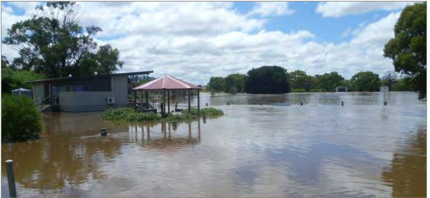
Figure 34. Shelford Recreation Reserve Oval impacted by flooding during the 2011 flood event (source: Jessica Myer).
