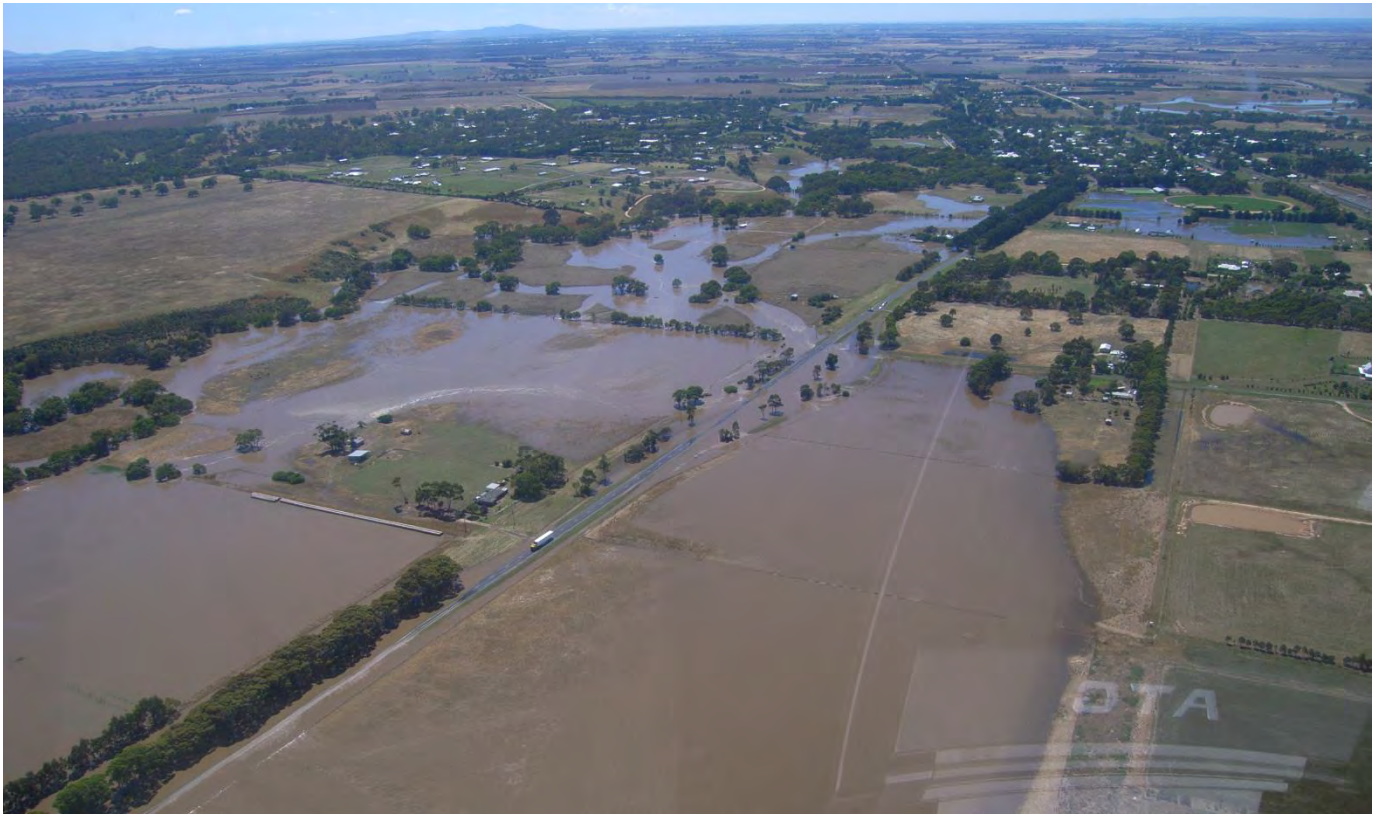
Figure 13. Flooding impacting the Hamilton Highway, looking east towards Inverleigh during the 2011 flood event.
