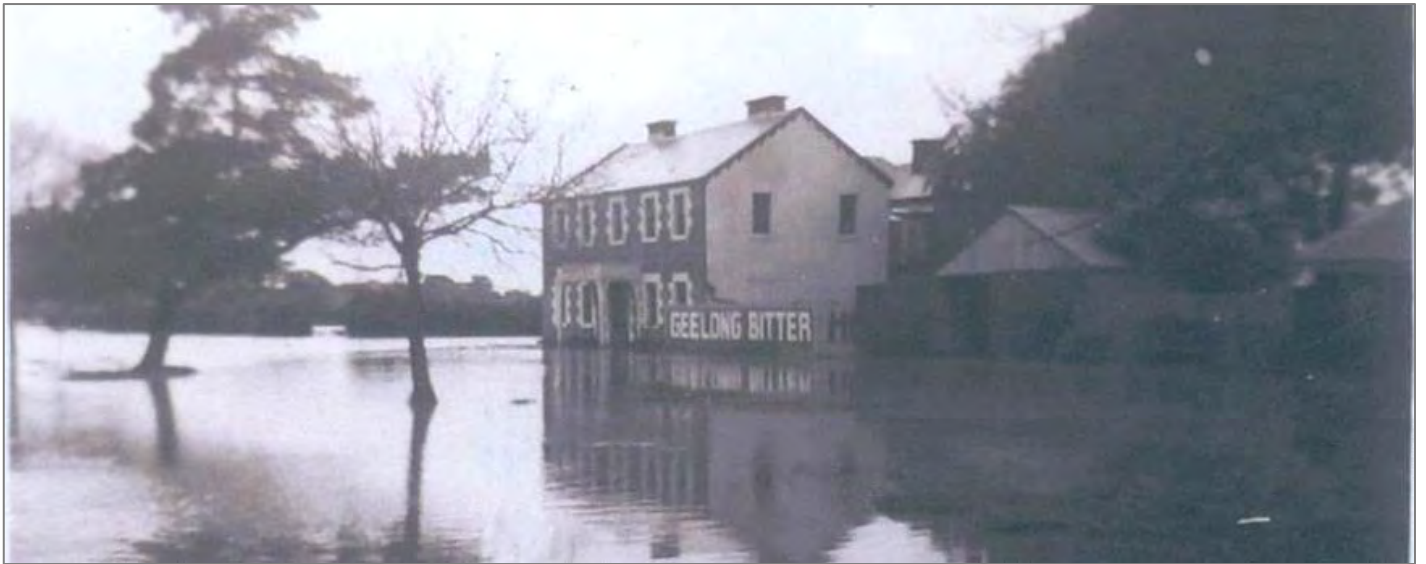
Figure 11. Flooding impacting the Inverleigh Hotel, 1 High Street during the 1952 flood event.
