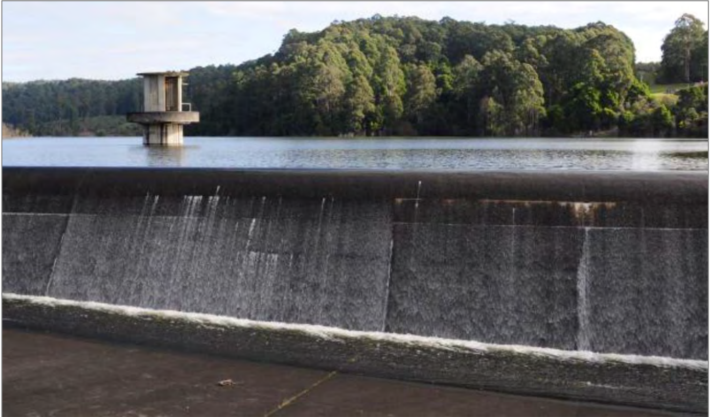
Figure 3. West Barwon Reservoir spillway.
