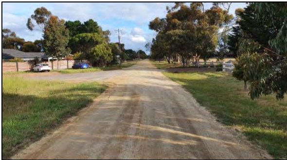
Figure 5: Ormond Street view Southeast
