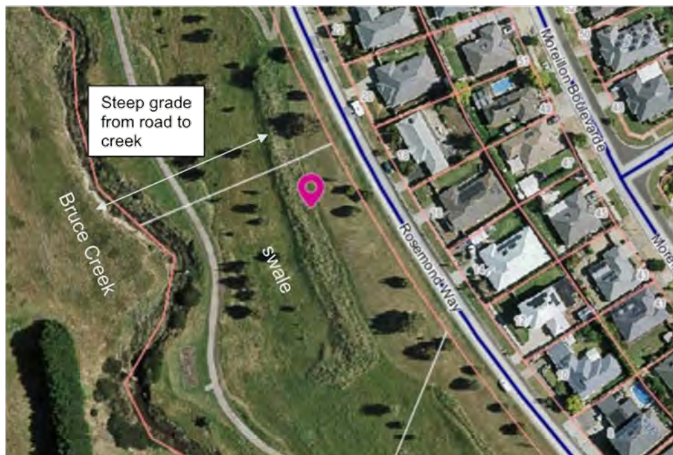
Figure 20: A vegetated swale that is inaccessible for maintenance activities due to the cross-sectional grade of the asset
