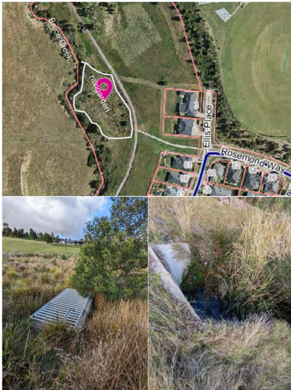
Figure 21: A stormwater raingarden basin with dry inlet and wet outlet to Bruce Creek.
