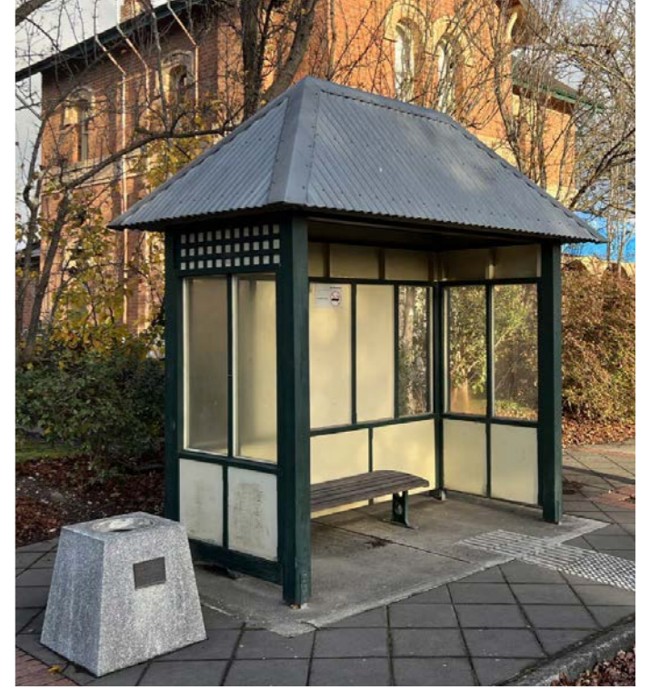
Bus shelter upgrades including relocation of shelter repair and repainting.
